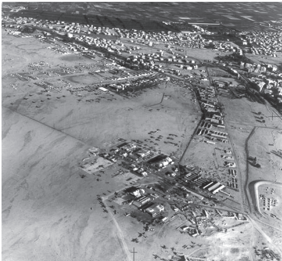
The RAF base at Heliopolis in 1942. The base did not have paved runways. The flat, hard packed sand was the landing field. Heliopolis was transformed over the years into what is now Cairo International Airport.
